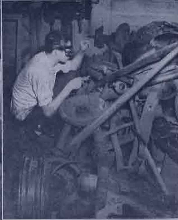
STILLMAN POND, welding shop
